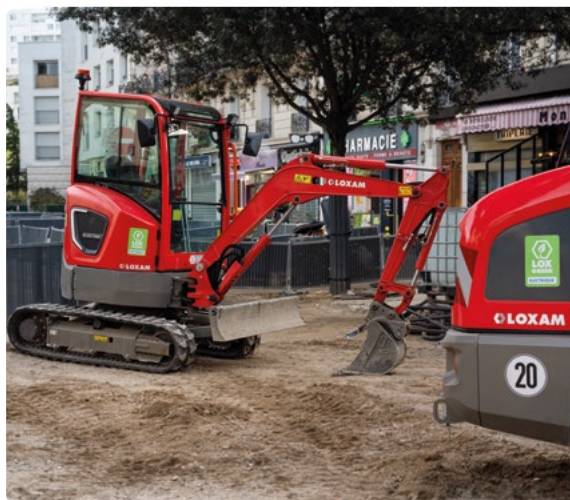
Example of a low-carbon construction site
